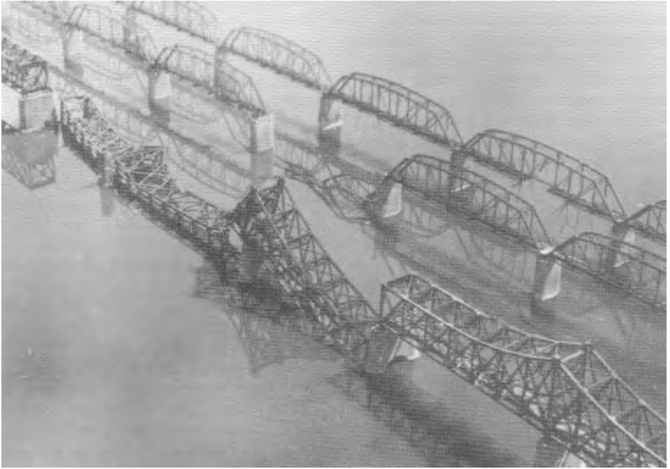
Reconnaissance photos prove the "elastic bridge" is sunk, 29 August 1950.
